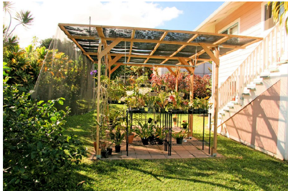
The finished structure
