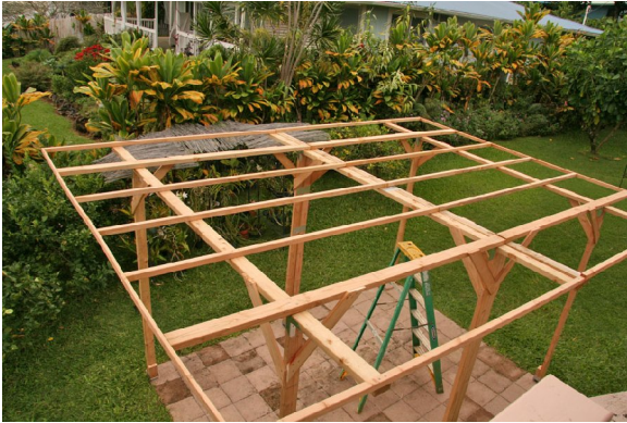
The frame under construction
